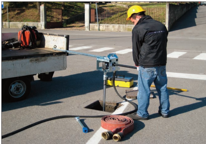
Picture shows "one man operation" with tool torsion force secured on a safe fix point
